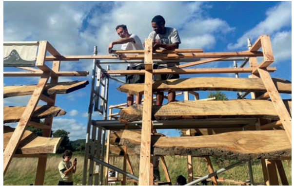
The Asker Meadows pavilion under construction
